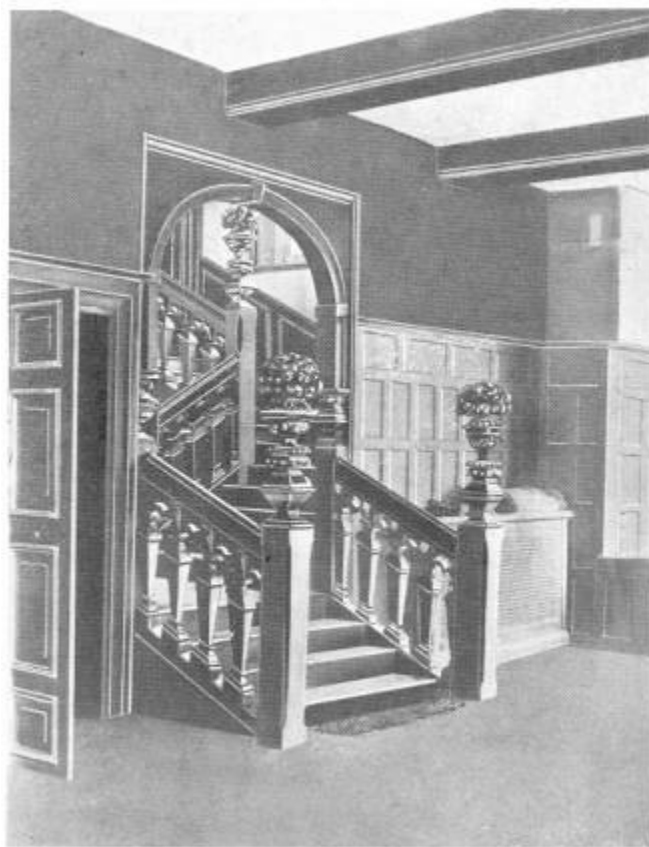
STAIRCASE, BROUGHTON HALL
