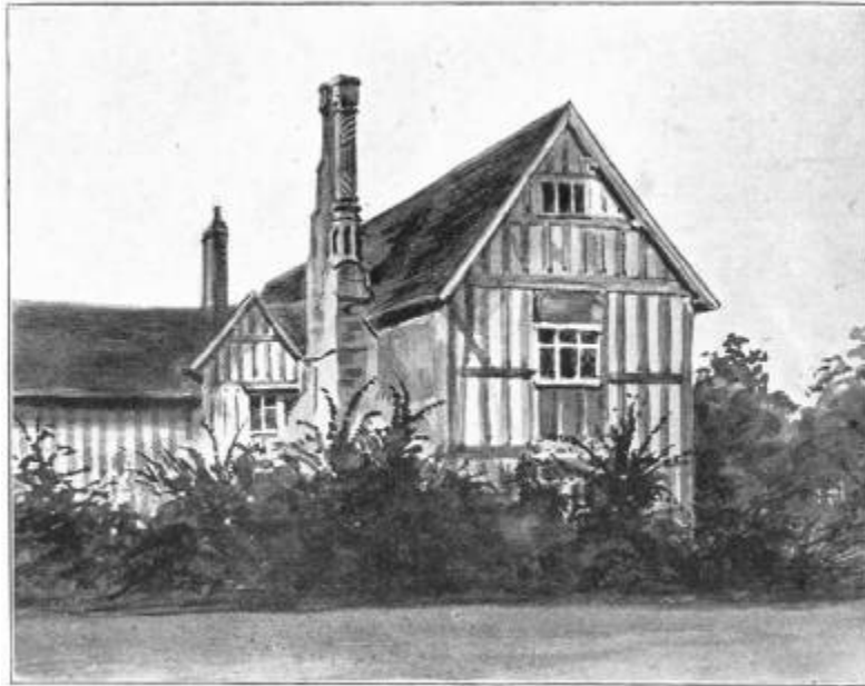
HUDDINGTON COURT, WORCESTERSHIRE
