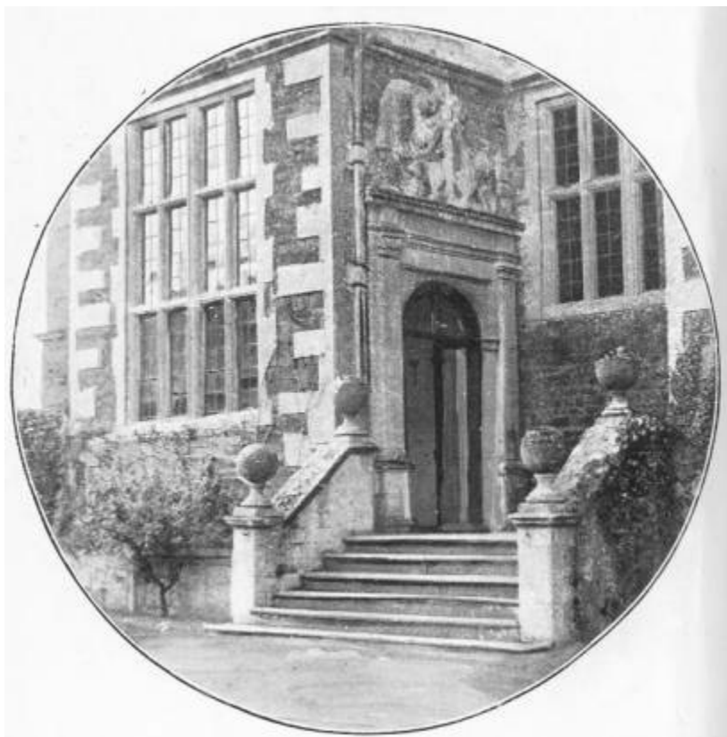
ENTRANCE DOOR, CHASTLETON
