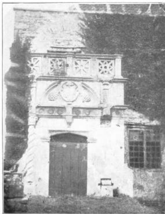
PORCH, CHELVEY COURT, SOMERSETSHIRE
