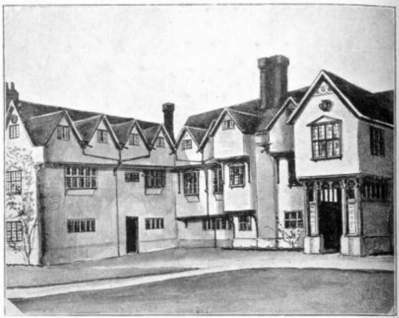
UFTON COURT, BERKSHIRE
